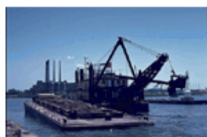
Dredging in wetlands or nearby waterways
