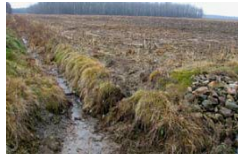
Erosion at the confluence of a ditch and a watercourse Source: Mikael Guillou ( MAPAQ )
